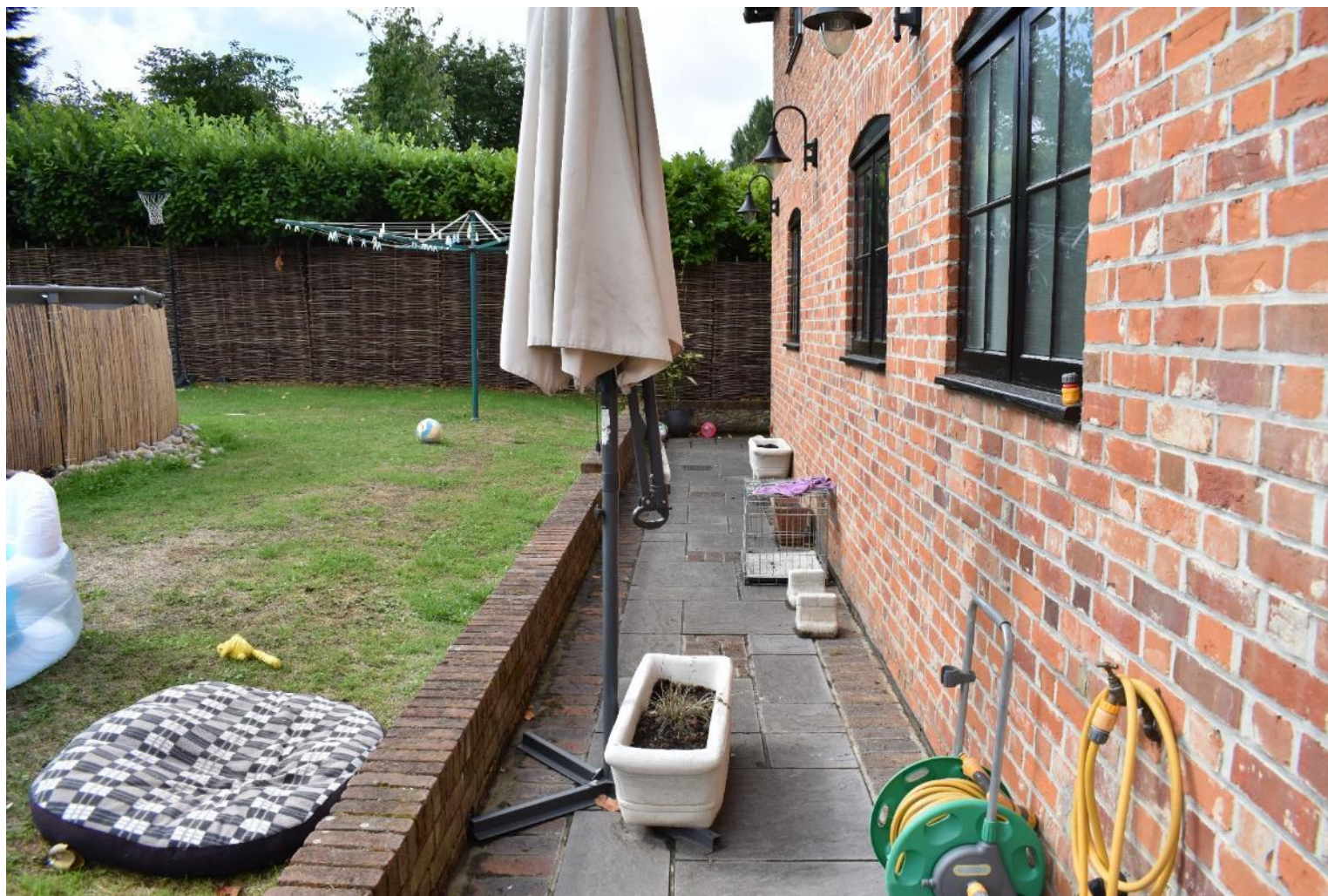
Plate 10: View of the retaining wall (facing S).
